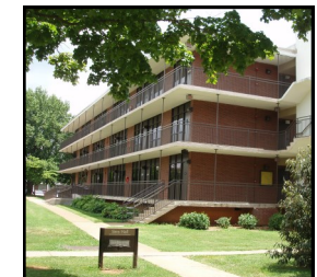
MTSU, Smith Housing Complex Murfreesboro, TN
